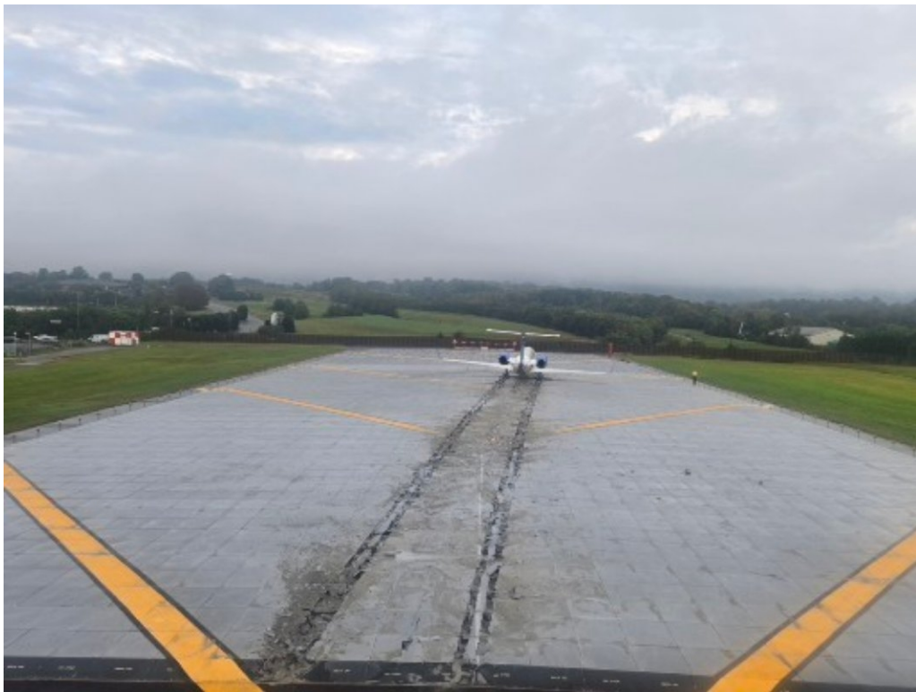
Figure 2. Airplane main landing gear witness marks in the EMAS at ROA. (Source: ROA)
